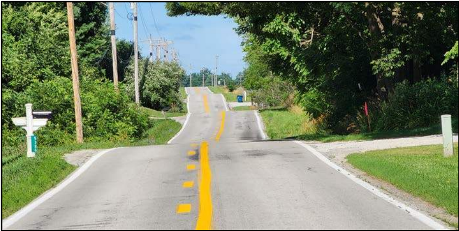
Narrow section view of SR 16 with 9’ travel lanes
