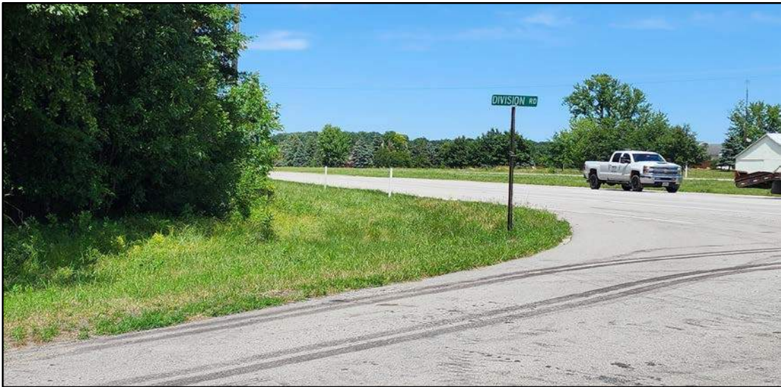
Sight distance obstructed for drivers looking north from Division Rd at SR 9
