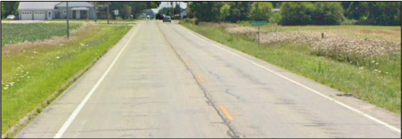
Existing section of SR 5 with 12' travel lanes and 2'-3' shoulders
