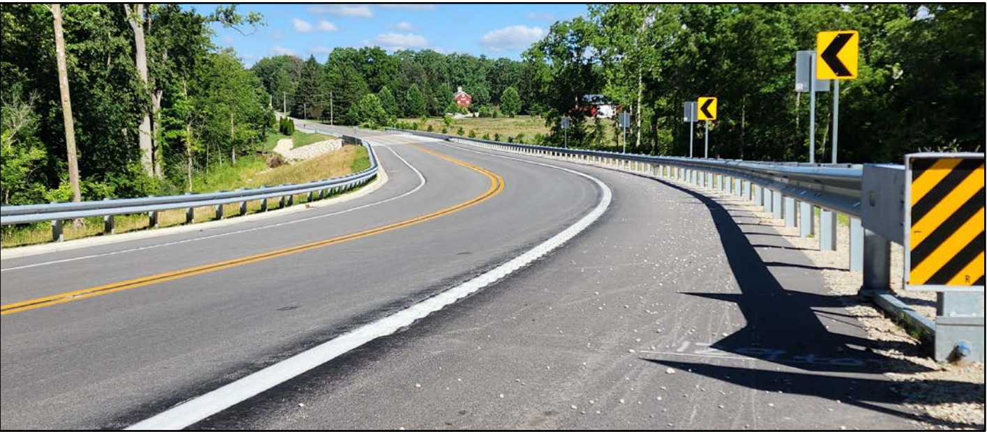
Widened SR 5 bridge and approach over Clear Creek to 12’ travel lanes and 5’ shoulders, completed in 2023
