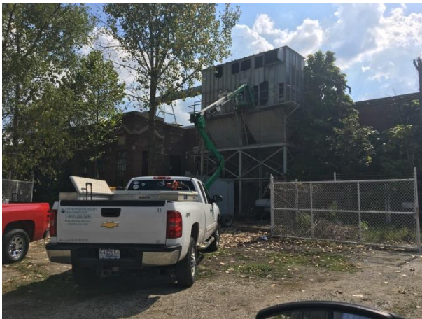
Workers from Quality Environmental Solutions, a United States Environmental Protection Agency Contractor, clean out one of the several dust collection baghouses at the former H.K. Porter site so that it may be removed during an earlier phase of the cleanup.
