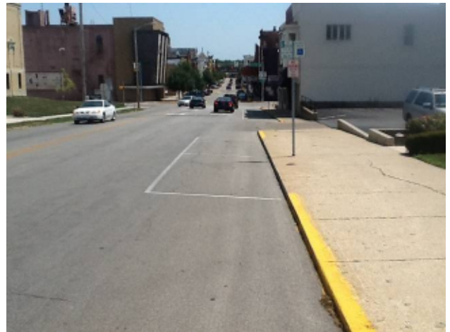
Photo illustrates on-street parallel parking on Jefferson St. Parking space slopes would make it extremely difficult for wheelchair user.
