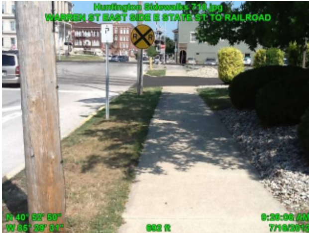
Photo shows typical condition at rail crossings within City for crossing with compliant slope but no detectable warning.
