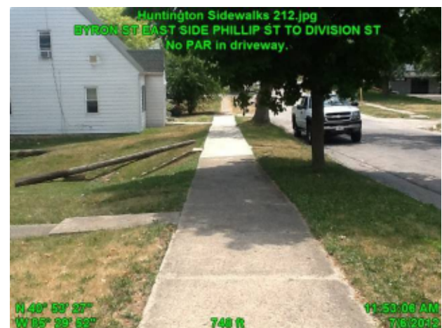
Photo: Example of 5' sidewalk width
