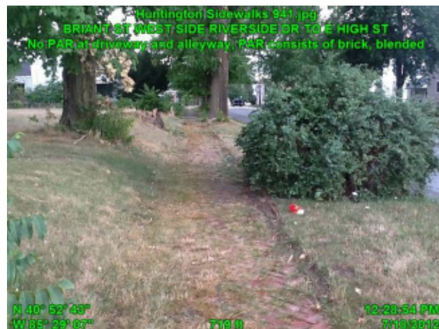
Photo: Example of poor surface (brick) that has not been maintained and has extensive areas of vegetation, which are surface level changes and present a difficulty for a wide variety of users.
