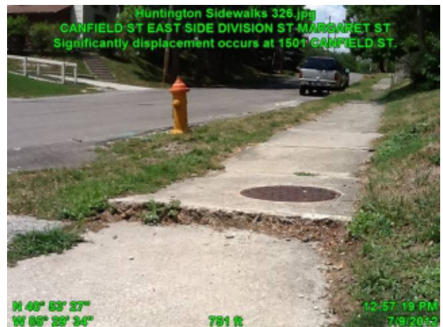
Photo: Example of ground plane utility conflicts as displacement and slip/trip hazard
