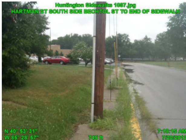
Example of Utility Obstruction narrowing sidewalk width to under 48" minimum required
