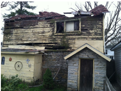
Garage Demolished in 2013
