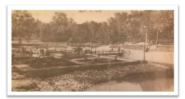
The Waltonian Garden water feature should be fully evaluated prior to being rehabilitated. Rehabilitation would likely include patching and sealing of all existing cracks, resurfacing with an appropriate waterproofing coating, testing and replacement of operable parts including controls and pumps, and adding drainage provisions where necessary to help maintain the life of the fountain with
